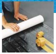
Without removing the "peel-off" from the tape, position the flooring on the floor boards/floor panels. Fold back half of the flooring, remove the "peel-off" from the tape and stick the flooring onto the tape. Please make sure no "air bubbles" are trapped underneath the flooring. Repeat for the remainder of the material.
