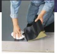
Install a wide, thin, self-adhesive protection tape onto the floor boards/floor panels. Let the tape "overlap", and install without "air bubbles".
