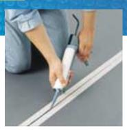
In order to make a clean seam, apply masking tape on both sides of the seam. After filling the groove with a sealant, smoothen as per the manufacturer's directions. Remove the masking tape.
