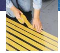
For final installation we recommend using a thin double-sided adhesive tape. For better results it is recommended to degrease the surface again. Distance between the individual strips of tape should be about 1 inch.
