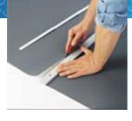
Cut the flooring to size, allowing 2 inches on each side, cut the exposed web edges. If possible seams need to be avoided in high traffic parts of the covered area. Cut the material outside of the aircraft or use a separate cutting surface to prevent damage to the aircraft floor boards/floor panels.
